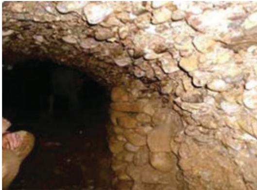
Discovery of drywalls in new tunnel sections
