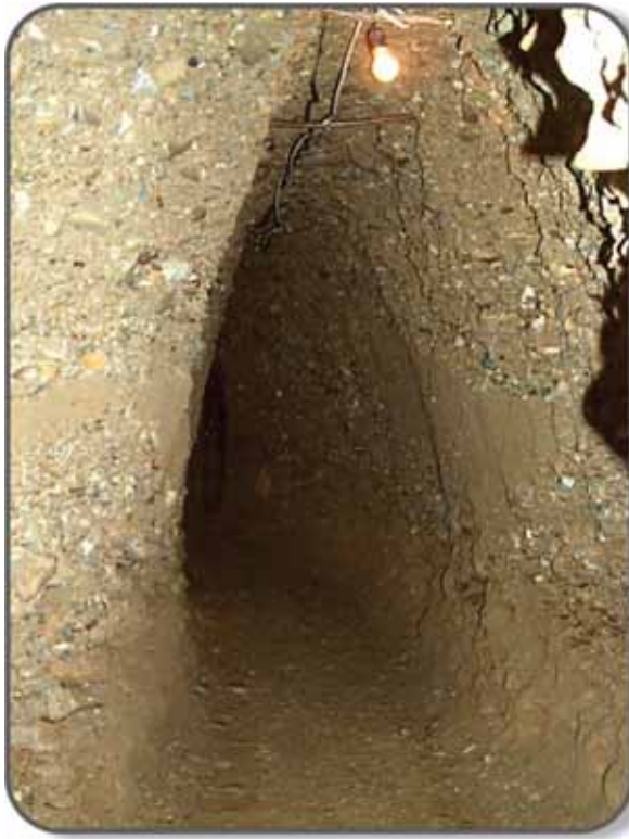
Tunnel section that leads to the first discovered gallery. This section is not secured by wooden supports because of it's structural stability.
