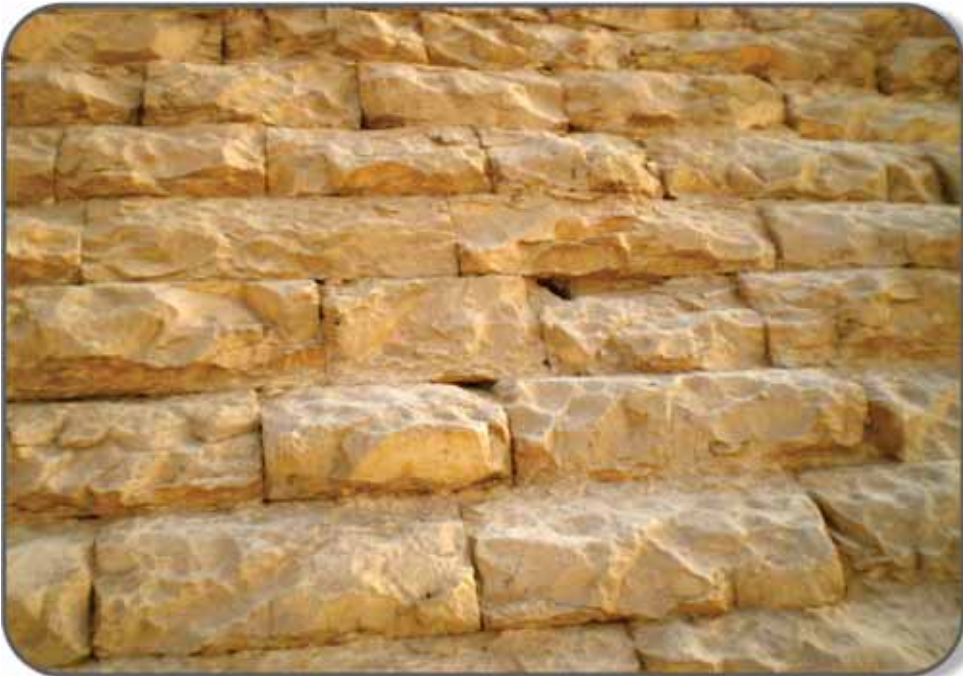
The reconstructed section of the outer layer of the pyramid in Meidum
