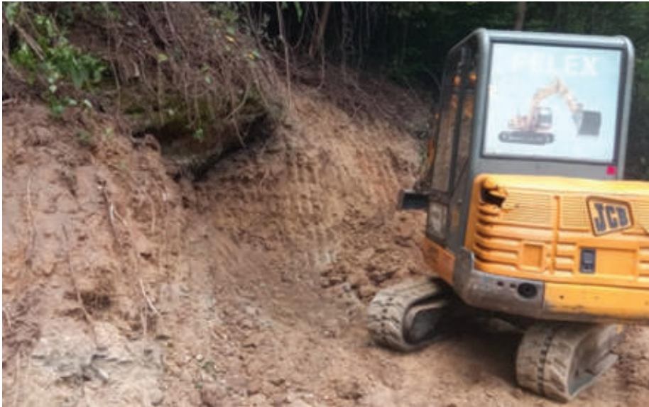
Photo 10; Earthworks being conducted in front of cavity 'C2', removing covering soil and marl layers beneath conglomerate exposure.
