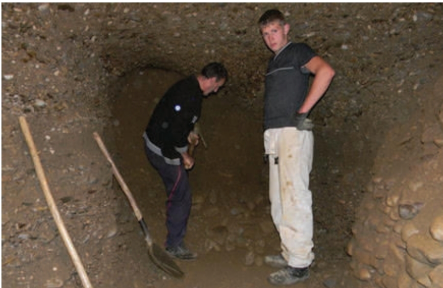
Photo 4; Ravne Tunnels being excavated in 2010. Loose rubble material being removed. A drywall construction retains material blocking side tunnel (right).
