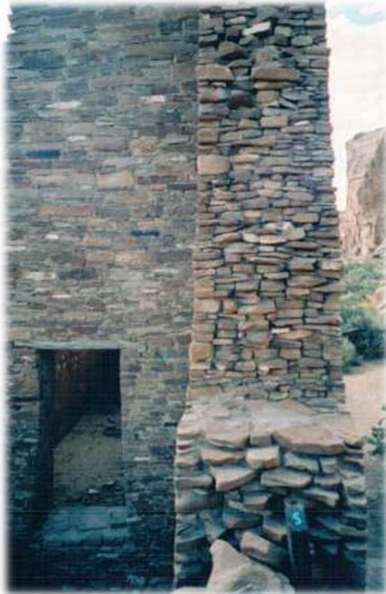
**Photo 12: The walls of Pueblo Bonito were carefully built with over 50 million carefully prepared stone tiles, Chaco Canyon, New Mexico.**
