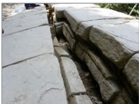
Figure 5(a): Close-up views of angular sandstone plates arranged in multiple horizontal layers.
