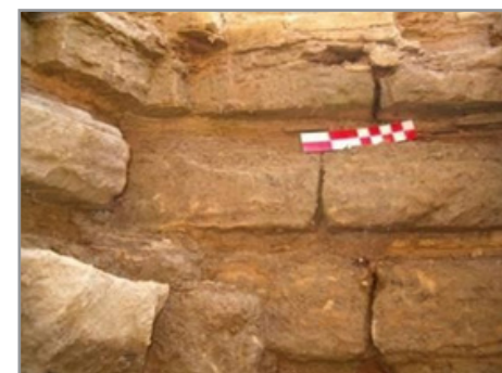
Figure 6(d): Stratigraphic profile showing alternating massive sandstone blocks and a layer of clay approximately ten centimetres thick, possibly serving as a binder and as thermal and acoustic insulation.
