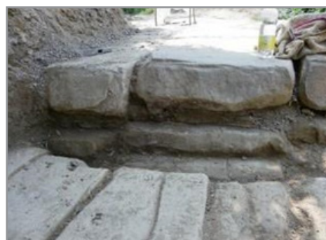
Figure 5(b): Close-up views of angular sandstone plates arranged in multiple horizontal layers.
